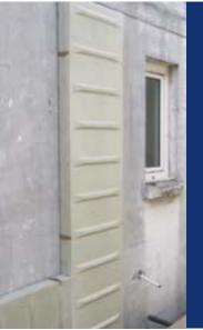
More than 320m of perforated GRP tray with standard covers was installed on the rear of the seafront hotel to hold air conditioning pipes and cables.
