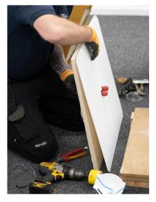
negotiating the pattress into the ceiling suspension system," says Daren. "It also allows us to work with a fire-rated material, compared to the traditional plywood or MDF pattress."
